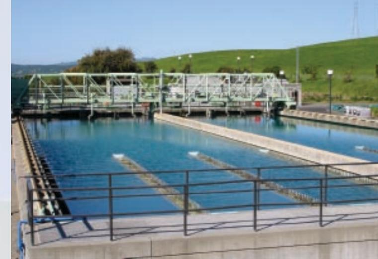
Drinking water is "settled" in a sedimentation basin at the Waterman Treatment Plant.
